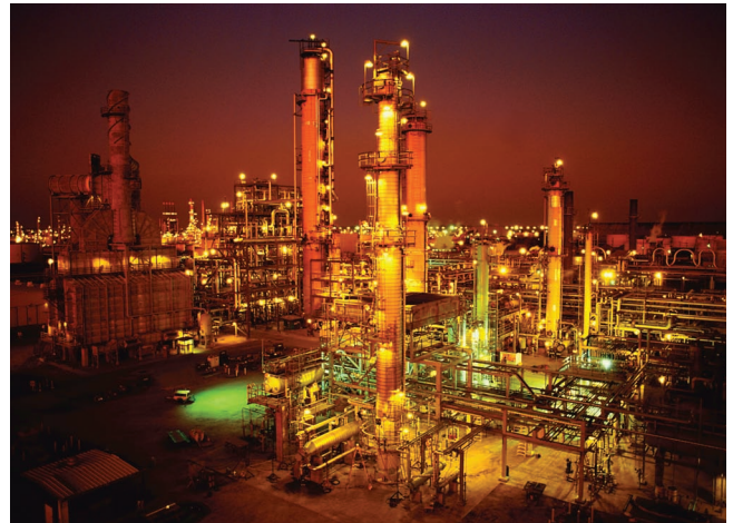
A continuous process: An oil refinery performs a continuous process, mixing and separating crude oil into gas, fuel oil, chemicals, and many other products.
